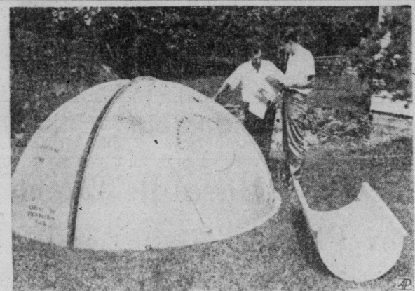
PLANS FOR SURVIVAL —Engineers for a bomb shelter manufacturer, Vincent Corubio, left, and Edward Klein, study specifications for a fiber glass dome shelter being installed on an estate in Locust Valley, N. Y. The dome is designed to cover an excavation, being dug in the background, which is to be floored, walled and outfitted for emergency living. (AP Wirephoto)
