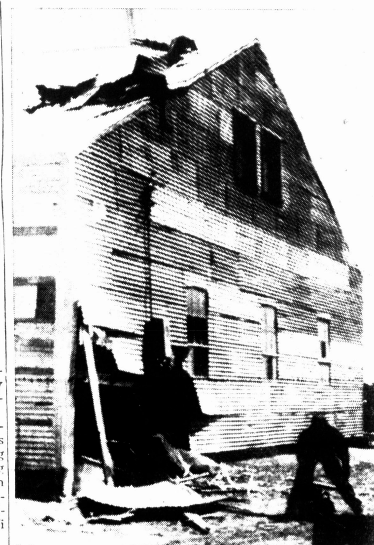
AIR COMPRESSOR EXPLODES — Flying pieces of metal pierced the roof and side of the Panhandle Auto Wrecking Co. building on E. Frederic after an air compressor exploded Monday afternoon. E. Frederic, manager, estimated damage at $1500. He said he thought the explosion was caused by a faulty safety valve. No one was injured. (News Photo)
