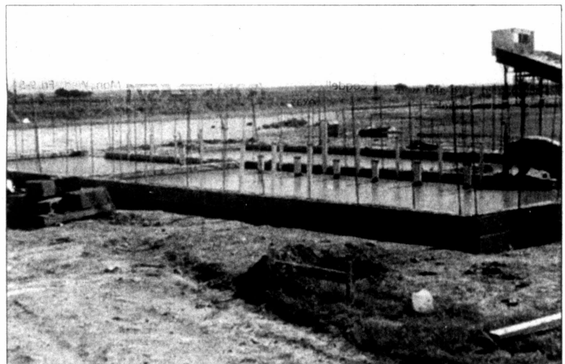
THE WESTBROOK WILDCATS get a new concession stand and restroom for the upcoming season which is just one of the new projects in the works.
