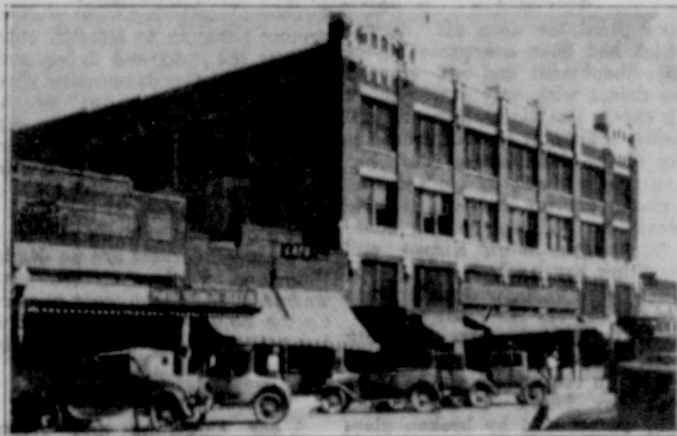
Above is shown a view of the Hodges-Neal Building, Ranger's best store building, recently purchased and remodeled to house the enlarged Joseph Dry Goods company, the formal opening of which will be staged Tuesday evening, Sept. 17. This picture was taken before the building was purchased by D. Joseph, owner of the store.
