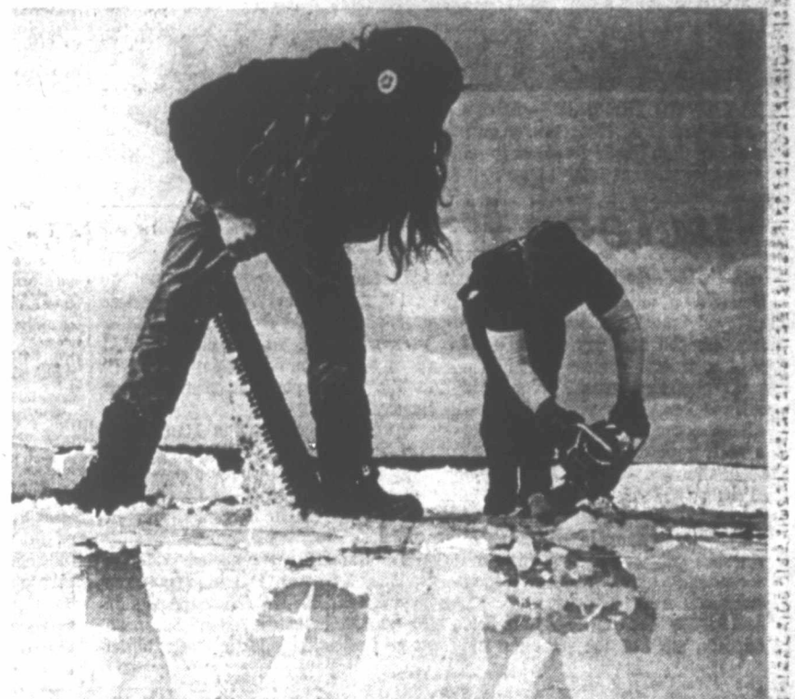
It takes an hour's work with 2 saws to cut entry hole in ice under snow.
