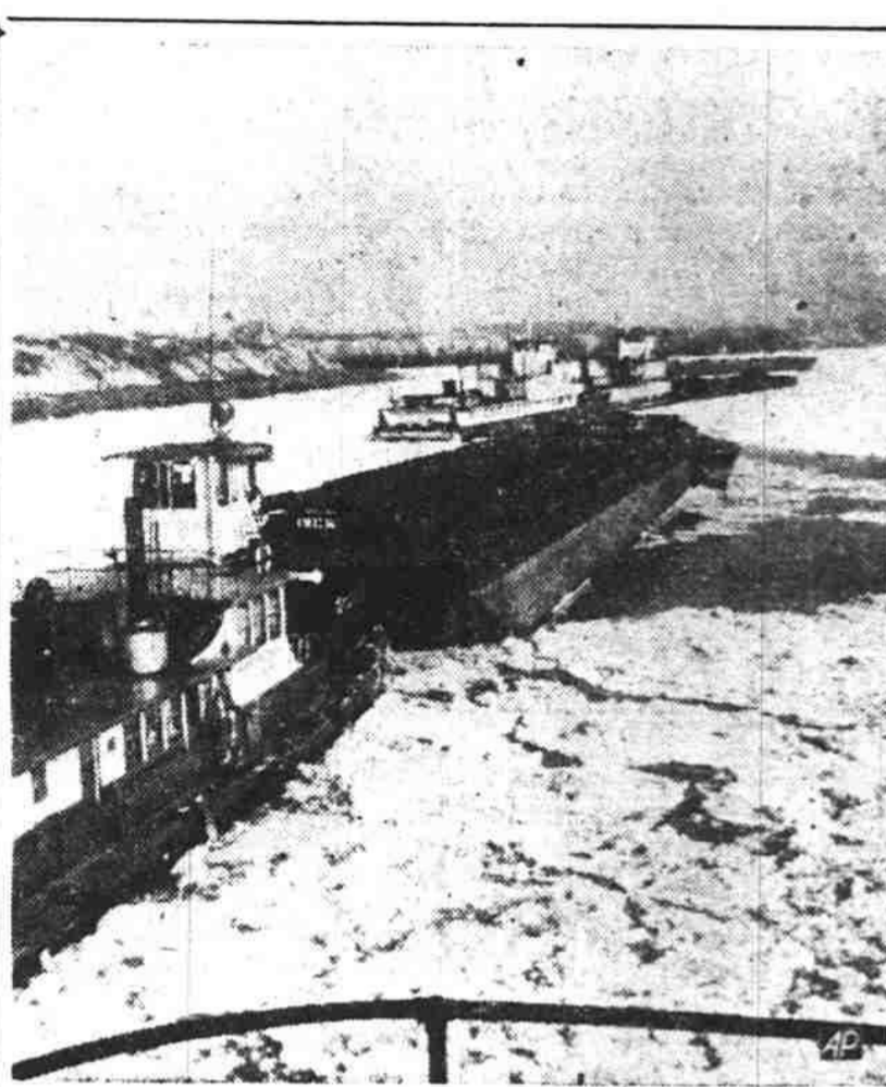
ICE-BREAKER WORKS TO FREE BOATS — An ice-breaker in front of a tug (foreground) chugs up the Illinois river near Ottawa, Ill., to release coal and oil barges (background), blocked by the heavy ice. The breaker had to keep on a continual move to free the boats and keep river traffic moving. (AP Wirephoto).
