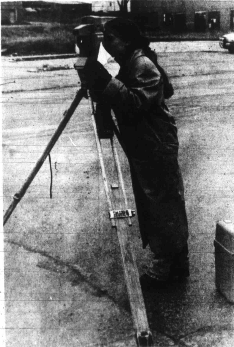
A REPRESENTATIVE OF STANLEY-MORRIS ENGINEERING out of Sweetwater was out in the cold Tuesday surveying parts of Colorado City for phase one of the city's pending water and sewer project.
