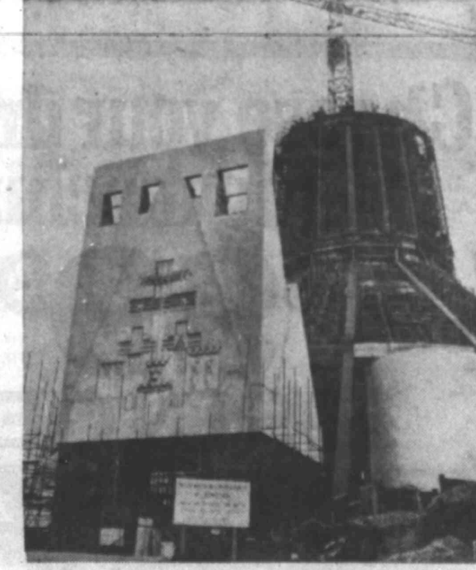
TAKING SHAPE — Erection of the Roman Catholic cathedral in Liverpool, England, continues. Entrance and nave are at left leading to the cone-shaped main edifice.
