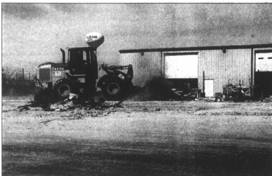
MAKING ROOM FOR SOMETHING NEW – The remnants of the Days Inn were being cleared away by heavy machinery operators last Friday. No plans of what will become of the property have been announced.
