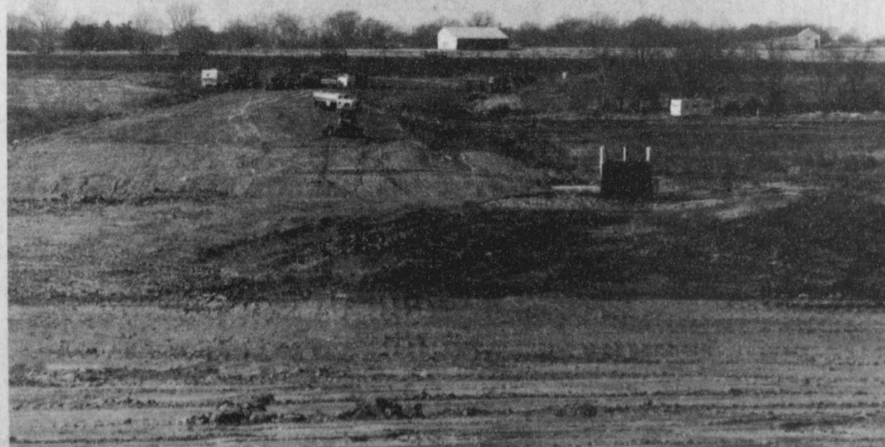
HEAVY equipment rolled to a stop because of the rain that soaked the soil
