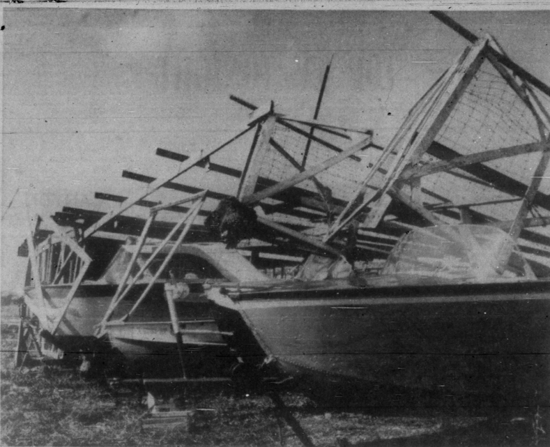
WIND DAMAGE AT LAKE THOMAS—Only one boat suffered minor damage as a freak wind demolished this boat house at Jinkins Grocery at Lake Thomas. High winds and large hail hit the area last night. Parts of the building were found as far away as the shoreline to the south and west.
