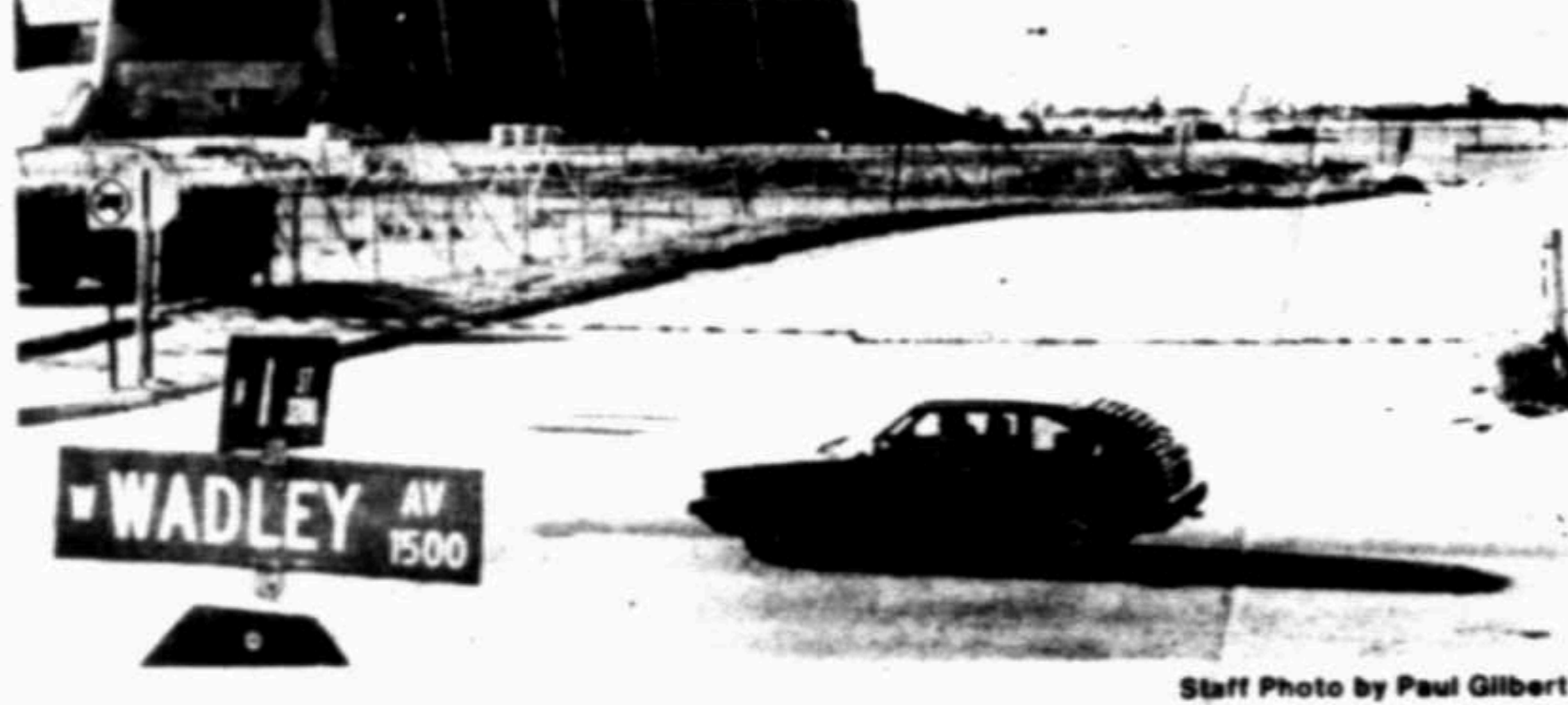
A gate to Midland College will swing open when a bridge is widened and a traffic light installed at the intersection of North I Street and Wadley Avenue.
