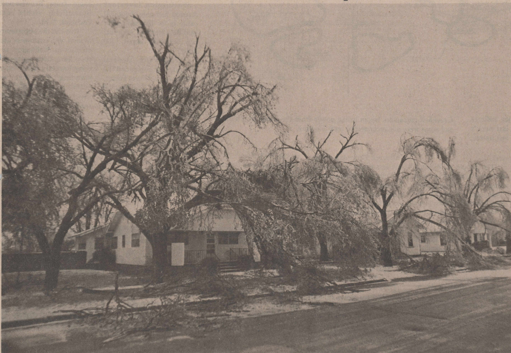
BROKEN TREE LIMBS... Elm trees around the Cal Sugg home lie broken and in the street after the worst ice storm in the county's history.
