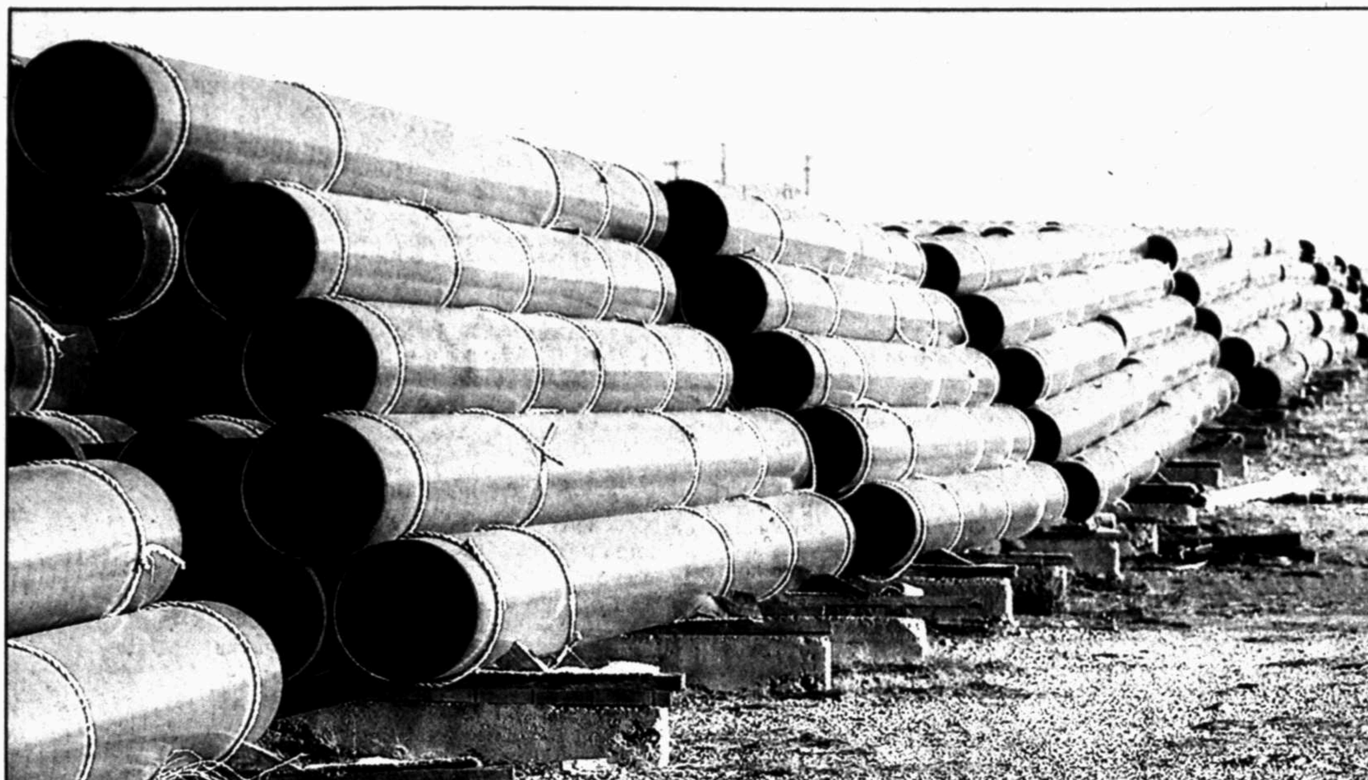
Miles of pipe stacked were stacked in an Odessa pipe yard this summer in preparation for construction of the Longhorn Partners Pipeline. The
