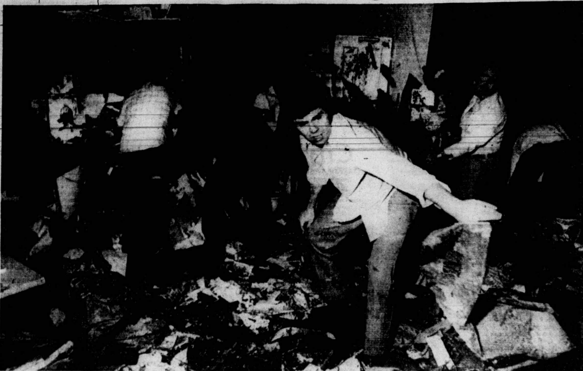
Volunteer rescue workers in Wichita Falls search through rubble of a small church destroyed by tornado that hit the city Tuesday night
