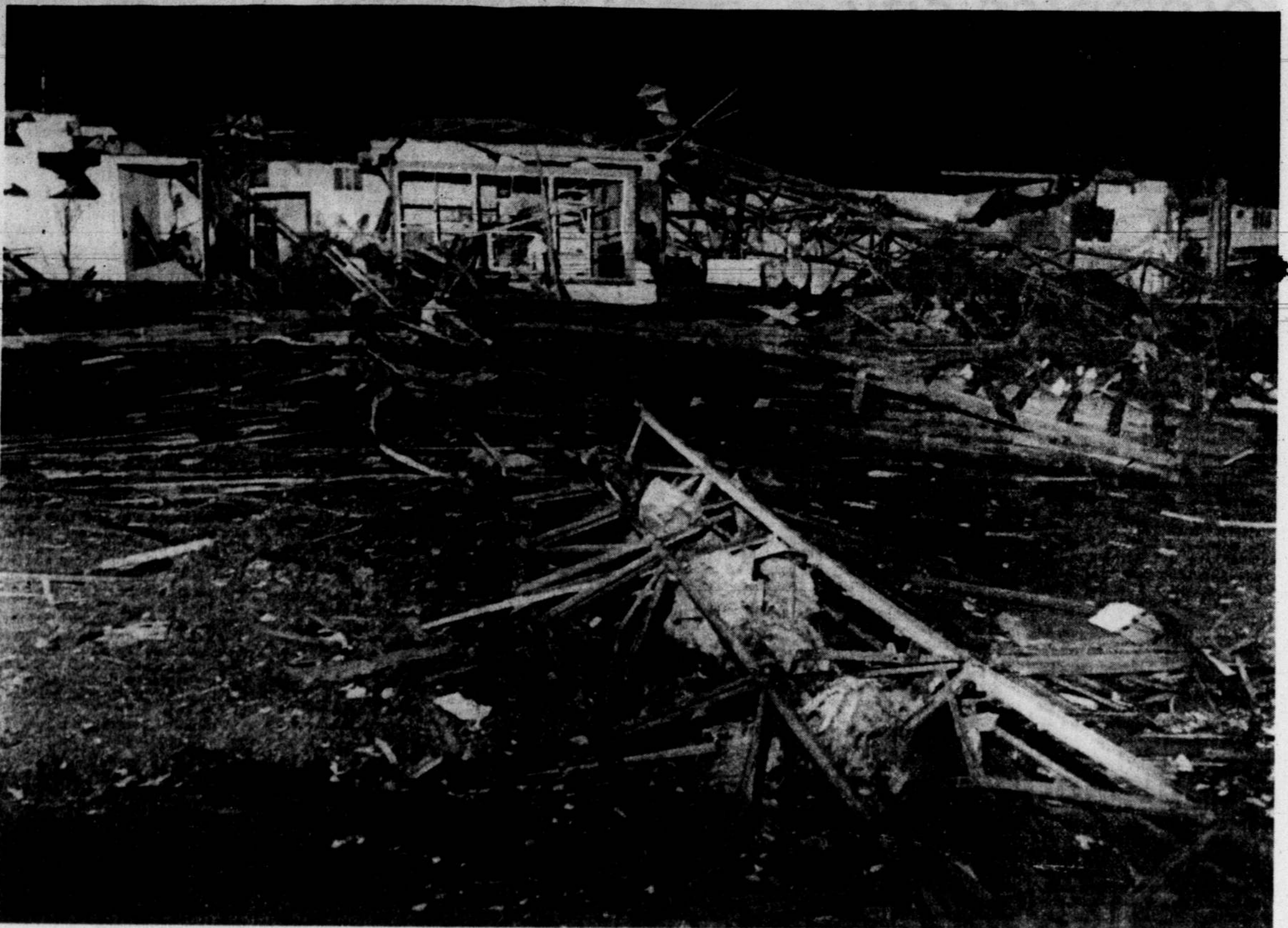
Shopping center sign becomes twisted wreckage 3 blocks away after twister
