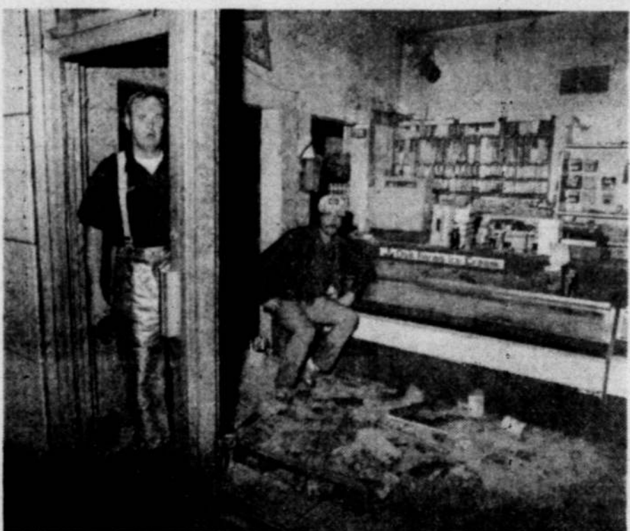
Wichita Falls firemen were on duty in damaged areas to help prevent looting of businesses Tuesday night.
