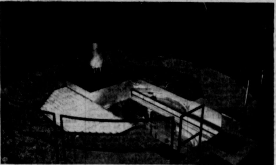
NUCLEAR PULSE REACTOR—The U. S. Army Ordnance Corps' first Nuclear Pulse Reactor was dedicated Oct. 17 at Walter Reed Army Medical Center, Forest Glen, Md. Nicknamed DORF—for Diamond Ordnance Radiation Facility—the reactor will be manned and operated by personnel of the Diamond Ordnance Fuze Laboratories. The pulsing reactor can simulate many of the conditions encountered in a nuclear blast with safety to operating personnel. Radiation effects on selected Army items of equipment then can be analyzed without the blast and heat effect of an exploding bomb. The reactor was constructed by General Dynamics Corp., Calif.
