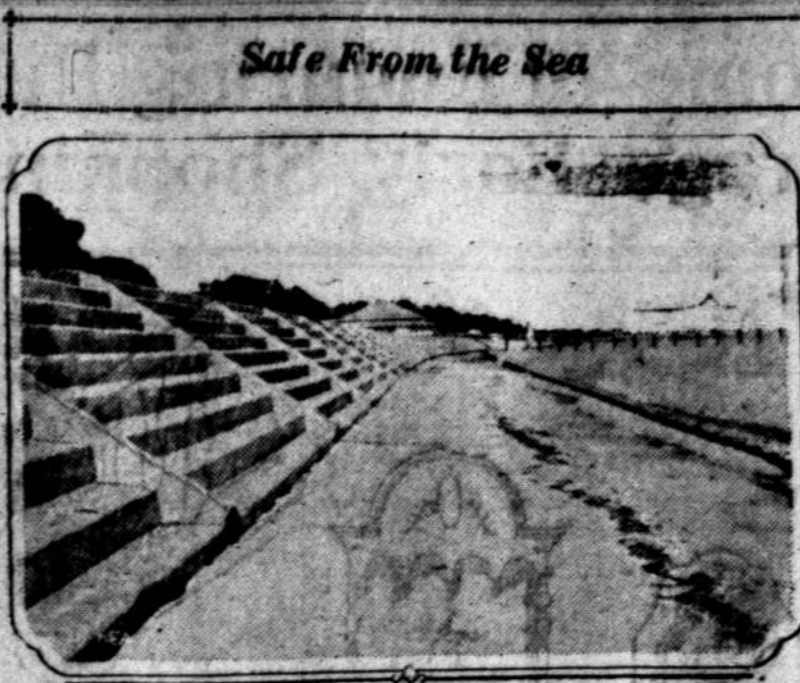
This concrete sea-wall is topped by a concrete stretch of the Old Spanish Trail along the Gulf of Mexico from Biloxi to Pass Christian, Miss. It is 24 1/2 miles long, and is said to be the longest sea-wall in the world. It cost $4,000,000 and will be completed in January.
