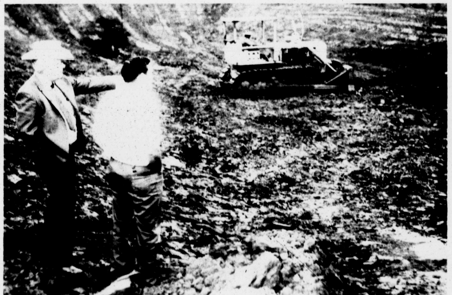
Reservoir Almost Finished
