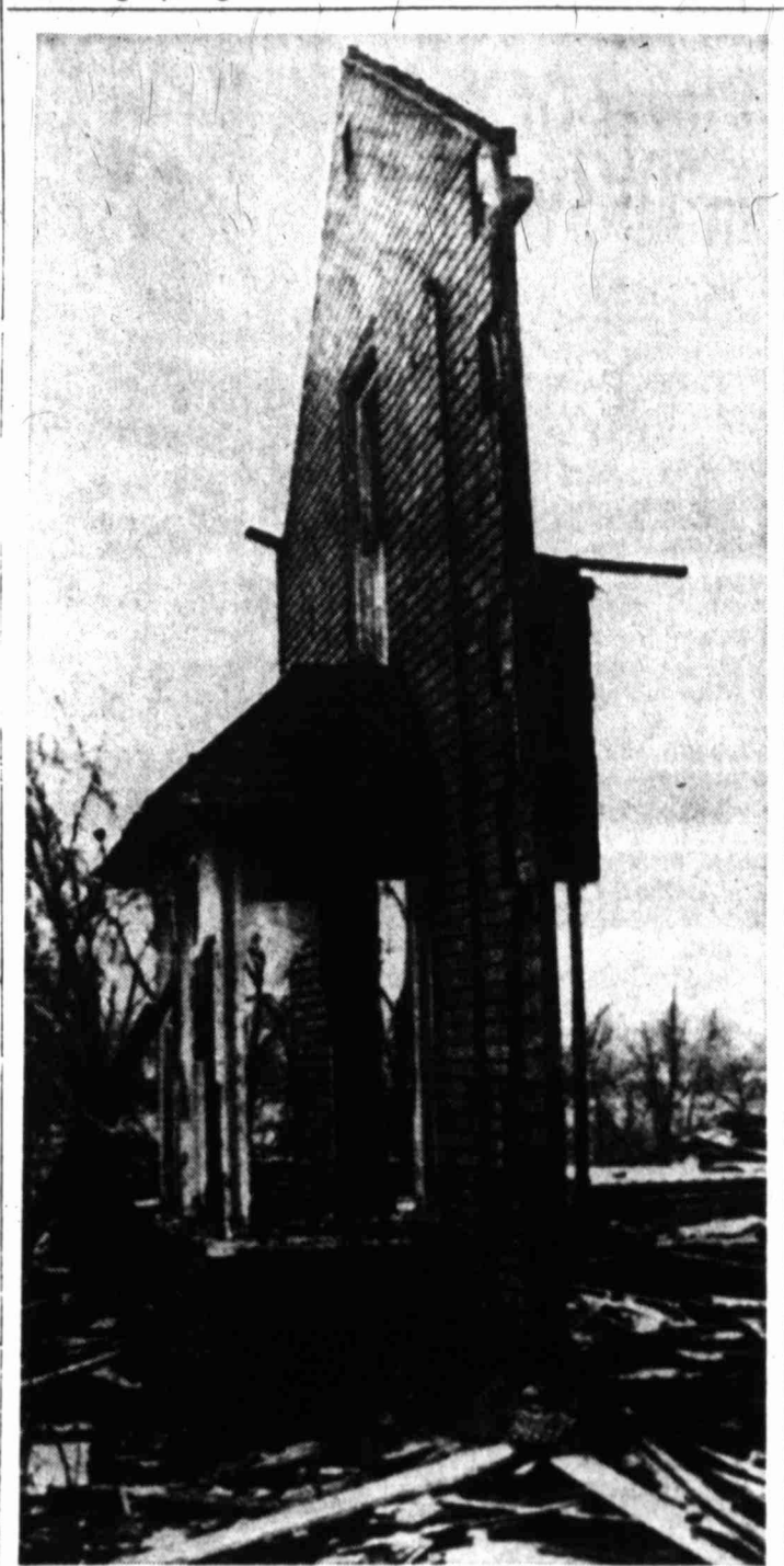
ONE SIDE OF STORY — Pisa has its leaning tower and Beloit, Wis., has its free-standing wall. It won't be there long enough to become a tourist trap, however, since it is destined for the wrecker's ball to make way for a parking lot.
