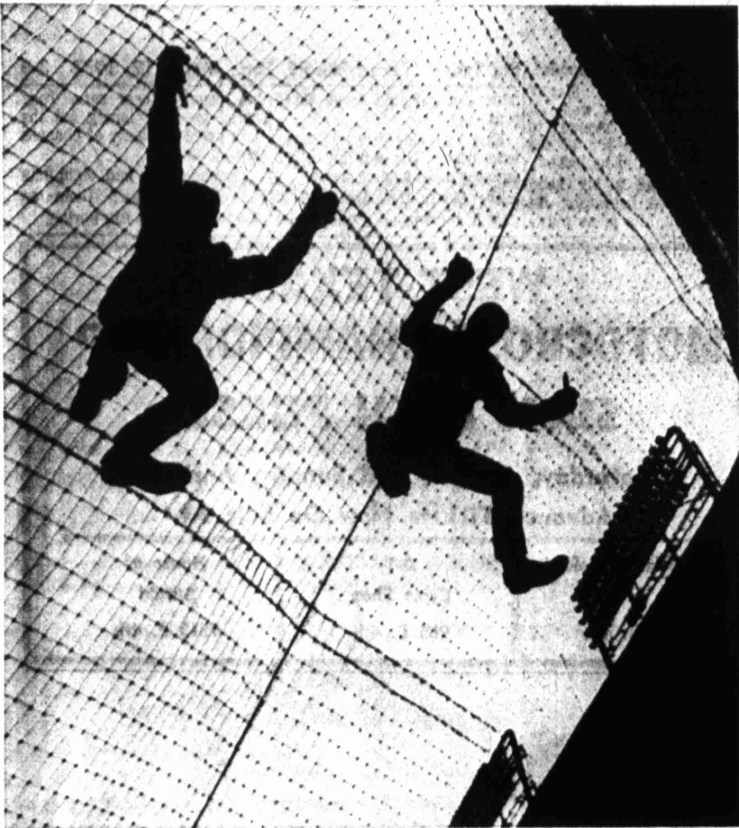
ONE MORE TIME — Workmen climb the steel screen behind home plate at Municipal Stadium to prepare for the home opening baseball game of the Kansas City Royals against California April 11. The job became necessary when it was determined the Royals' new stadium at the Harry S. Truman Sports Complex would not be ready until mid-summer.
