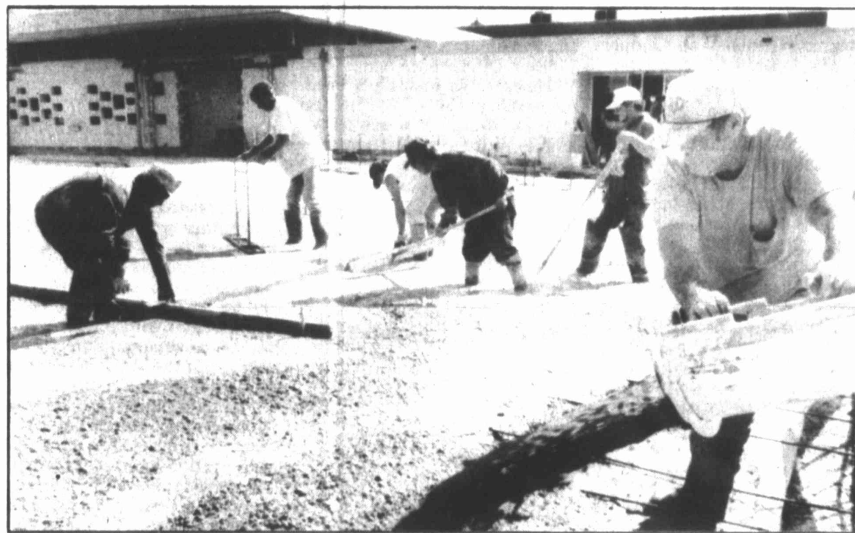
Workers smooth out freshly-poured concrete while more is poured into forms at the new Howard County Library Wednesday. The former Bluebonnet Savings building is being extended to the alley.
