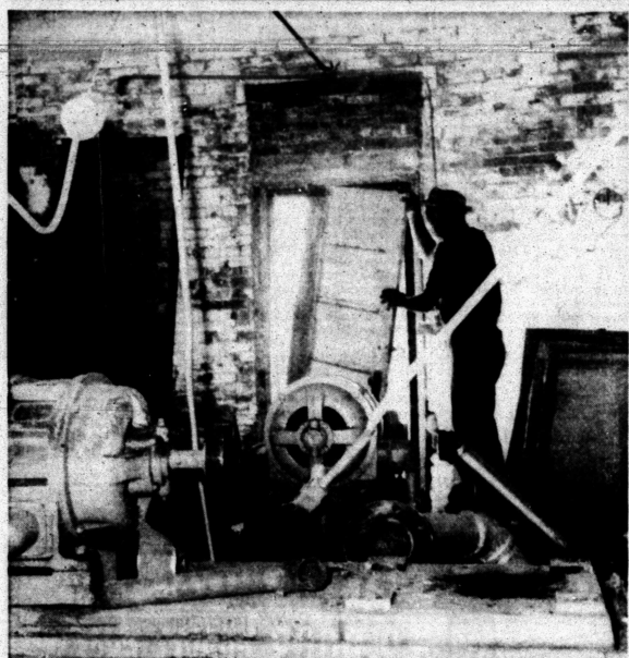
THE BEGINNING OF THE END for the old city hall building on west Twenty-sixth Street started last week as city employees began salvaging materials from an unused office at the east end of the building. That portion served as the water department when the building was built, and in the back of the office was this water well and pump which served the entire city of Snyder. In later years this area was the police station. City employee Bill Cooper is shown removing the back door to the room during the salvage operation.
