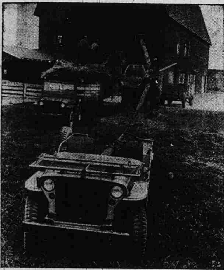
JEeps ON FARM —Two Jeeps, especially adapted for peace-time use, go to work in a farm demonstration. Vehicle in foreground serves as power unit for threshing machine, while Jeep in rear is ready to haul the wagon.
