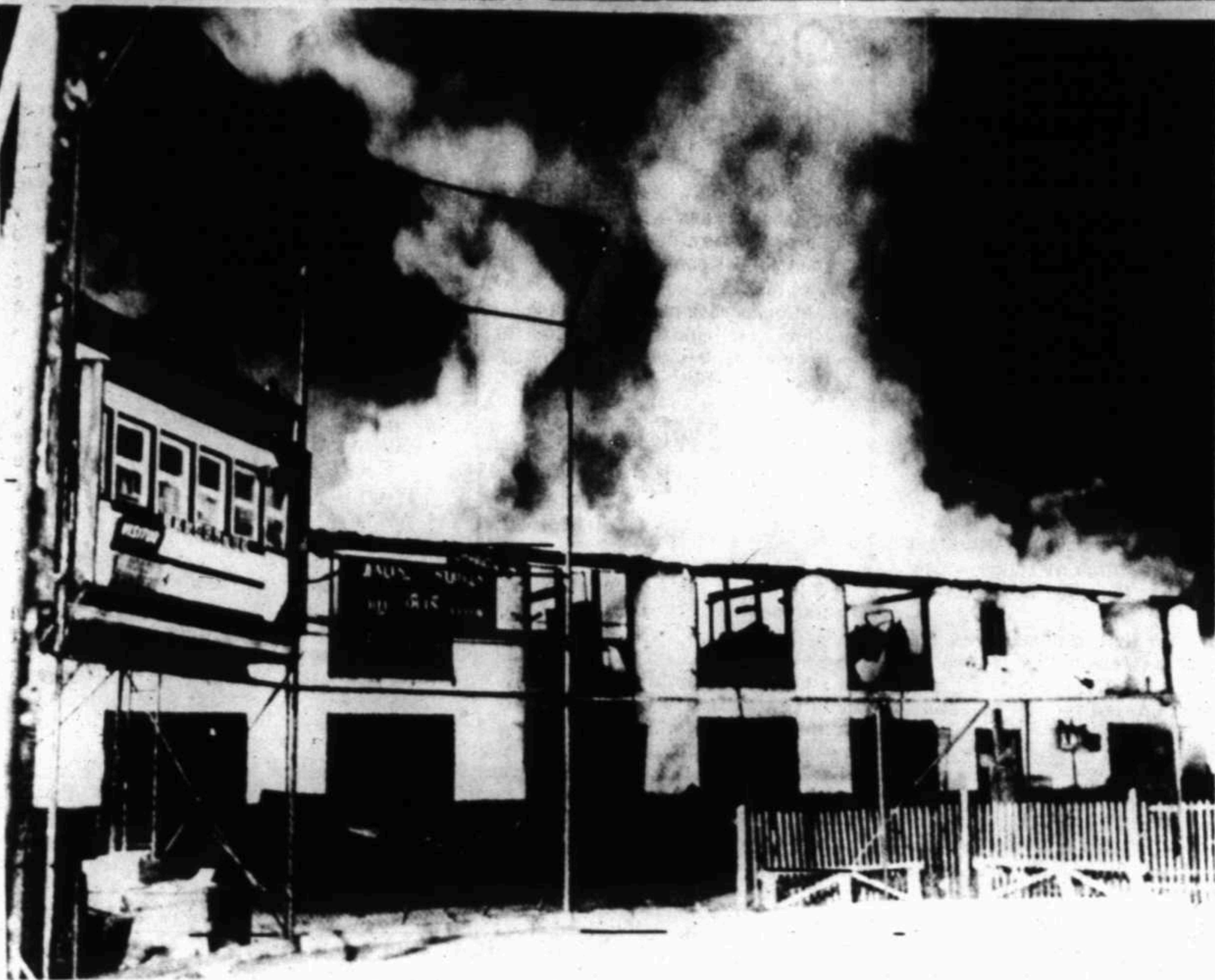
Buildings at Marquette State Prison in Marquette, Mich., smolder early Wednesday after inmates rioted and set fire to several buildings in the
