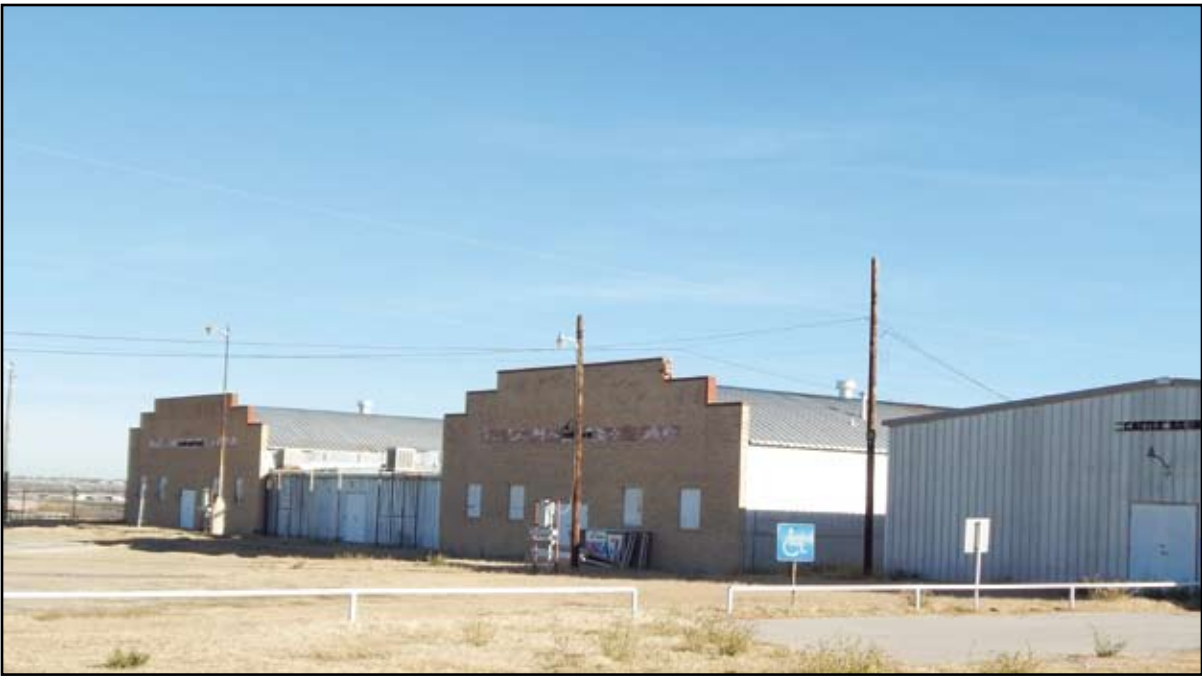
HERALD Photo/Andreia Medlin The Howard County Fair Show Barns are slated to be demolished according to officials. The decades old buildings have fallen into disrepair.
