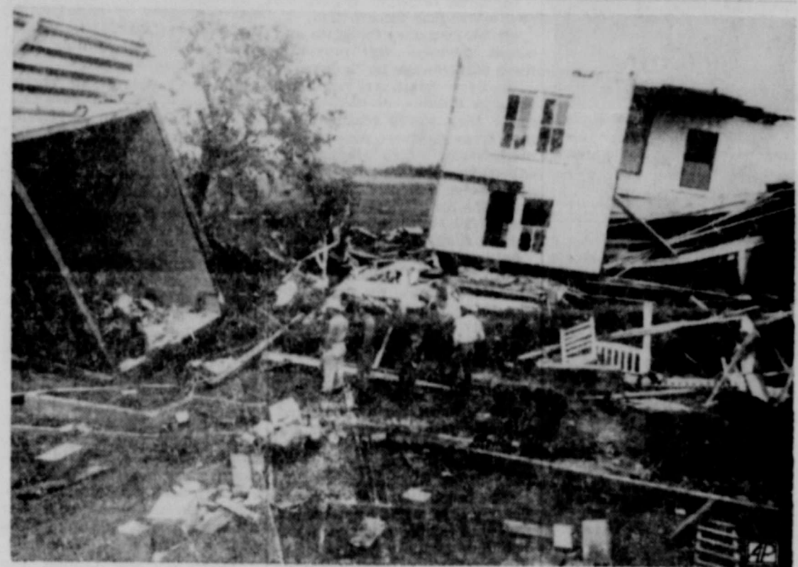
DEMOLISHED IN STORM'S PATH—Six persons were in the Otto Koerth home at La Bahia, 15 miles west of Brenham, Texas, when a tornado picked up the house, tore it in half, and threw one of the pieces end-over-end. The doors were blocked or high in the air, forcing the occupants to escape by window. Miraculously, no one was hurt seriously, but livestock were killed in the yard. The storm damaged nearby houses and barns to a lesser extent. (AP Wirephoto)
