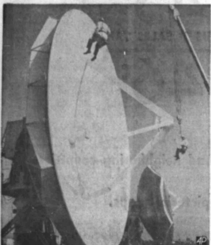
SPACE TRAPEZE —Men in bosun's chairs adjust saucer-like antenna of Mark 1B terminal which will link ground with satellites launched for global communication.
