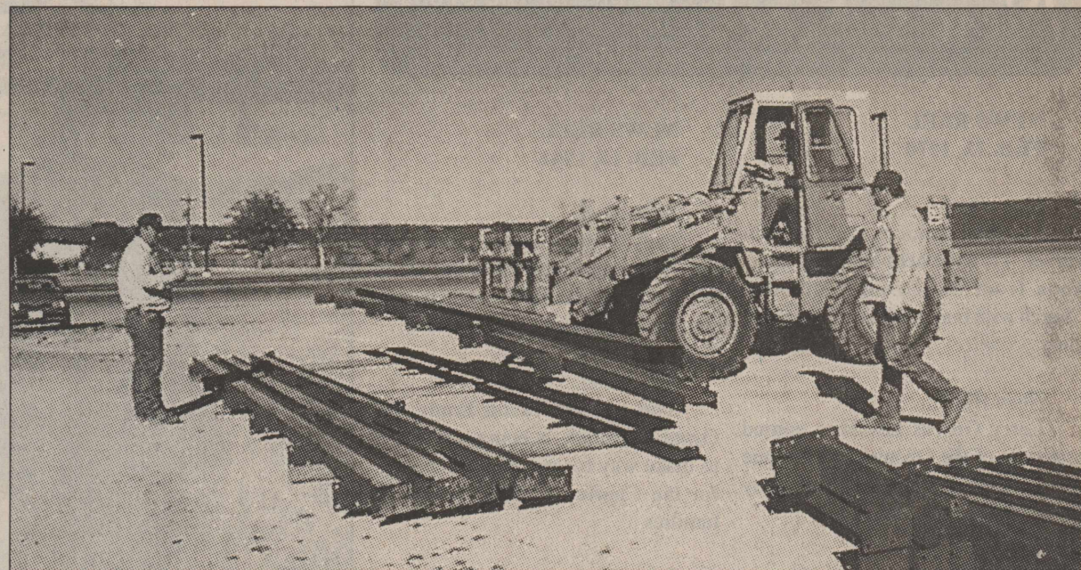
EDDIE MOORE (l.) and Ray Elkins direct backhoe operator Richard Sanchez as building materials from Metco Supply of Junction are unloaded. Construction of the Ozona Senior Citizens building is expected to begin this week.
