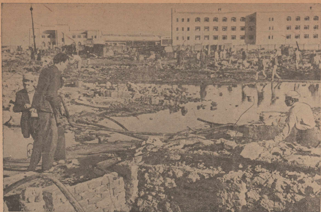
ERASING THE SCARS OF WAR —Egyptian workmen clear away the rubble of buildings smashed by the air and sea bombardment which accompanied the Anglo-French invasion of Port Said. The United Nations salvage fleet has resumed efforts to clear the blocked Suez Canal, of which Port Said is the northern terminus.
