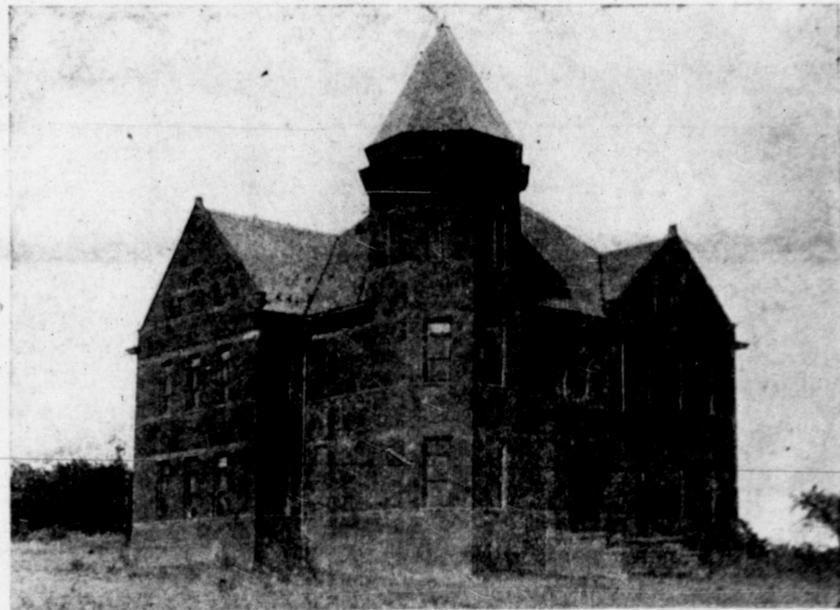
WARD SCHOOL BUILDING
