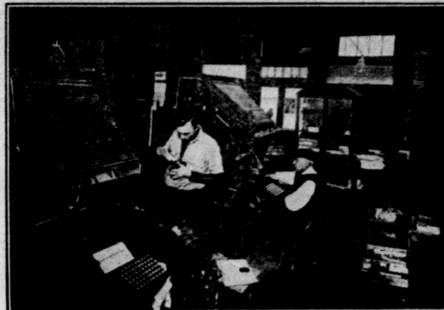
Interior view of Record office showing battery of Linotypes
