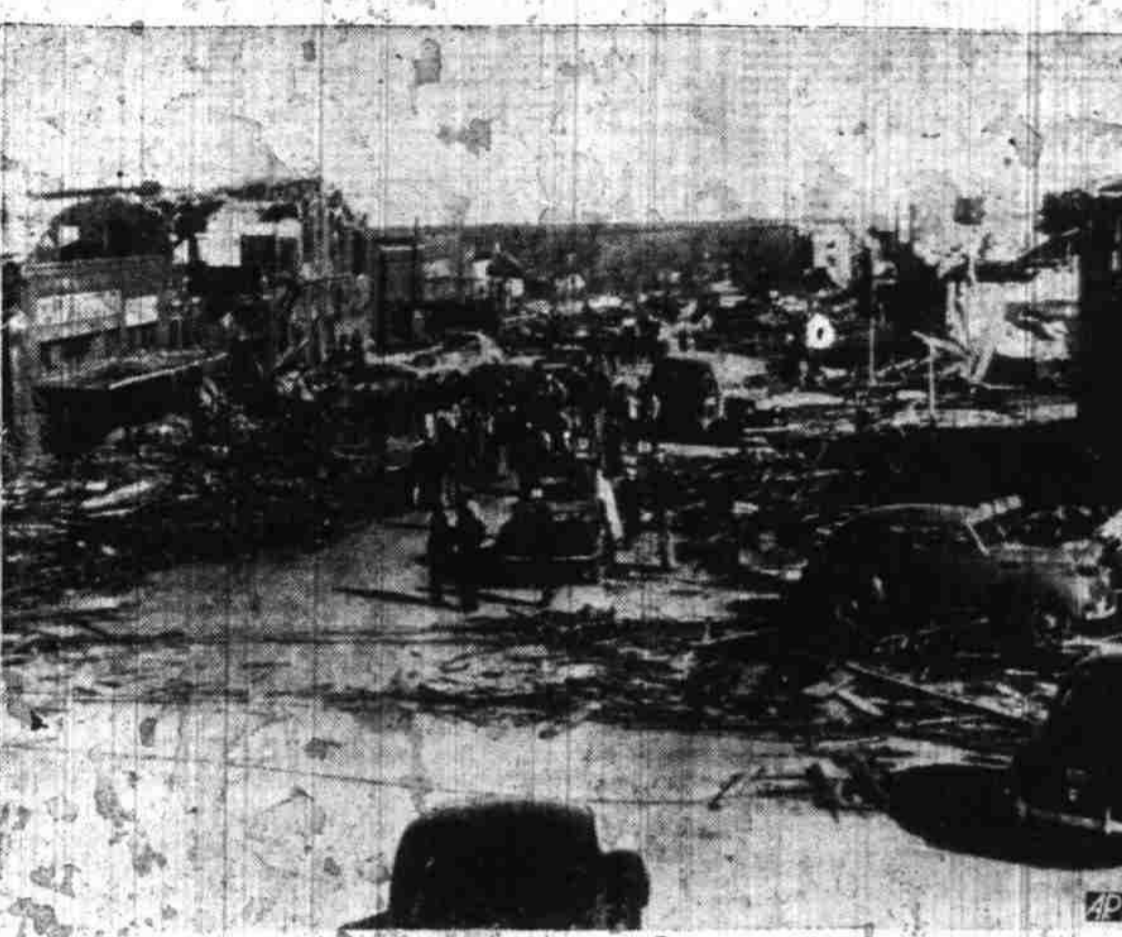
TWISTER FLATTENS HIGGINS, TEXAS—This is a view of the main street of Higgins, Tex., after a tornado which took a heavy casualty and property toll struck Texas and Oklahoma Panhandle towns. (AP Wirephoto).
