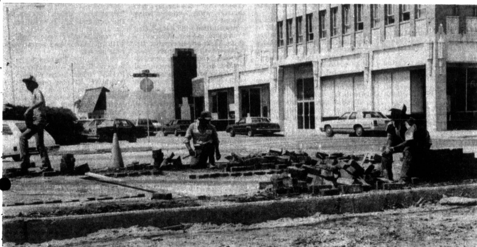
BRICKLAYERS — Workers show various degrees of energy as they put Kingsmill Avenue back together on the north side of City Hall. The construction on Kingsmill is part of
