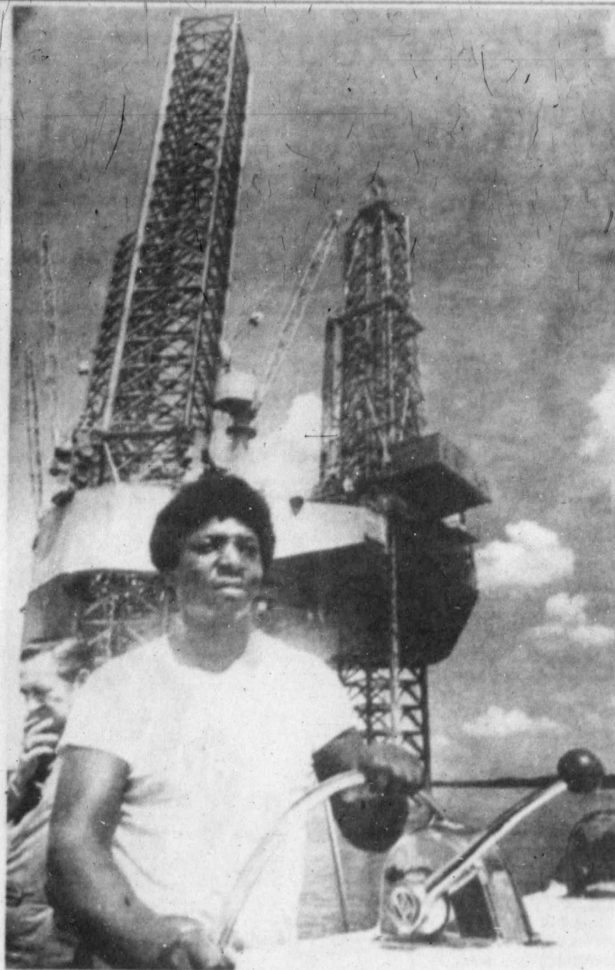
READY TO SAIL — A jack-up drilling rig rises against the sky in the background offshore New Orleans, with its three legs sticking into the air. Sails will be attached to the legs in a unique experiment to sail the rig to its site in the Gulf of Mexico. In the foreground, a small boat departs the rig, returning crewmen to shore.
