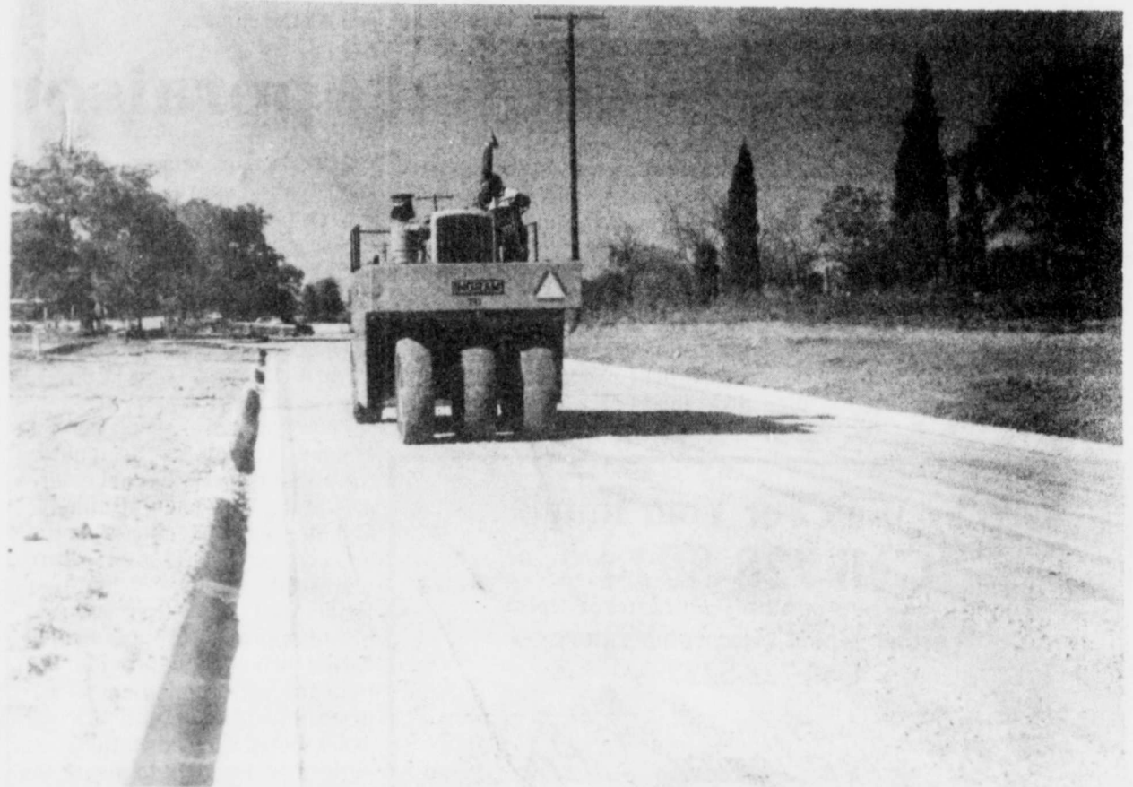
Construction crews prepare streets for paving
