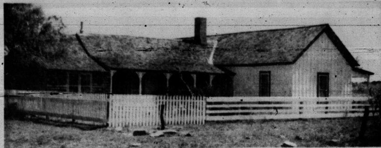
THIS PICTURE was taken Tuesday as Misses Myrtle and Faye Harrell wind up two years of hard work on the ranch home. The home includes six rooms, hall and bath.
