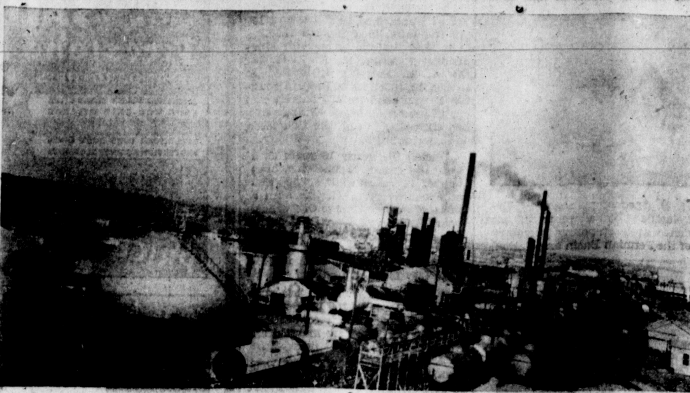
PARTIAL VIEW OF COL-TEX REFINERY
