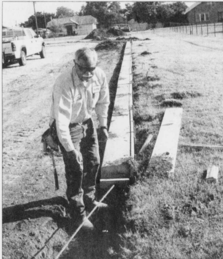
AND THE WORK goes on... Carlos Castaneda of Earthco pours curbing at the track at Hutchinson Elementary as part of Colorado ISD's campus update work. The track should be completed well before school starts in August.
