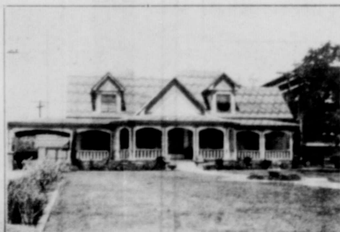
Above is the beautiful home of Mrs. Nannie Walker, on North Marston Street, which has recently been moved closer into town and remodeled.
