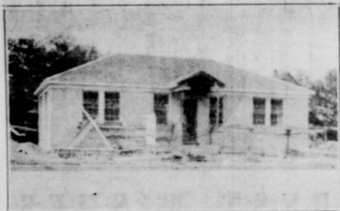
The new Ranger Clinic Building, which is now being constructed, will be occupied by Dr. W. L. and Dr. C. L. Jackson, upon completion. The building is a brick veneer of modern design. It is located on North Austin Street.
