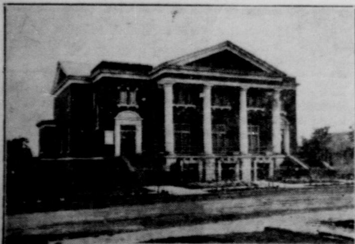
The First Methodist Church of Ranger occupies a beautiful brick building, which replaced the smaller, wooden structure the church owned prior to 1920.
