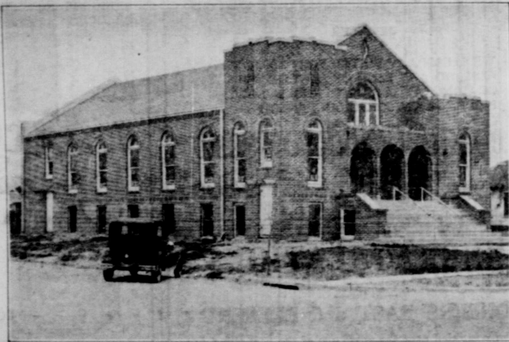
The beautiful brick Church of Christ building in Ranger is a monument to the determination of a congregation that needed a new building. Having only an old wooden building, in the depths of the depression, the modern brick building, pictured above, was built and paid for as it was constructed. When the new building was dedicated there was no outstanding indebtedness against the building.
