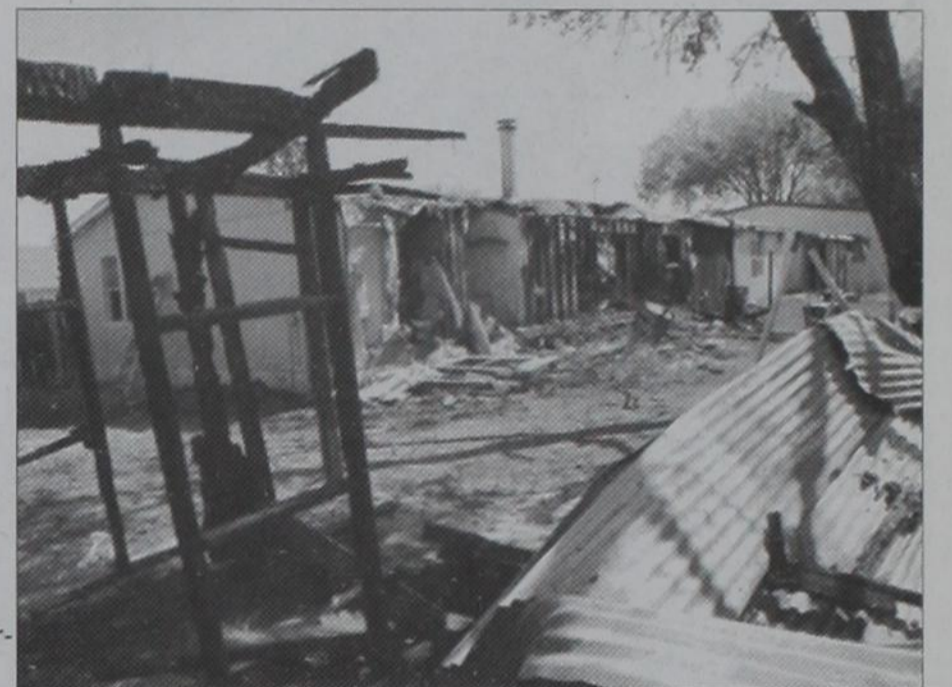
HOUSE FIRE: The Cathy Burrell home at 200 West Eighth in Wheeler burned Saturday afternoon. As the picture shows, it was a total loss. The building in the foreground was also a loss. Also the Wheeler Volunteer Fire Department was called to a grass fire just inside the state line Monday afternoon. The number of acres of lovegrass burned was not known at press time.
