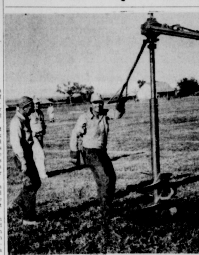
FOLLETT FIELD LIGHTS—George Symons and Carl Sward of Community Public Service are pictured above boring a hole for Follett's new field lights which are scheduled to be in use Friday night when the Panthers play their first home game against Sunray. Latest power equipment above enable the Community Public Service line-men to sink holes for the poles in a matter of minutes.
