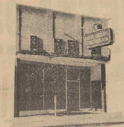
Recently remodeled WTU office at Clarendon
