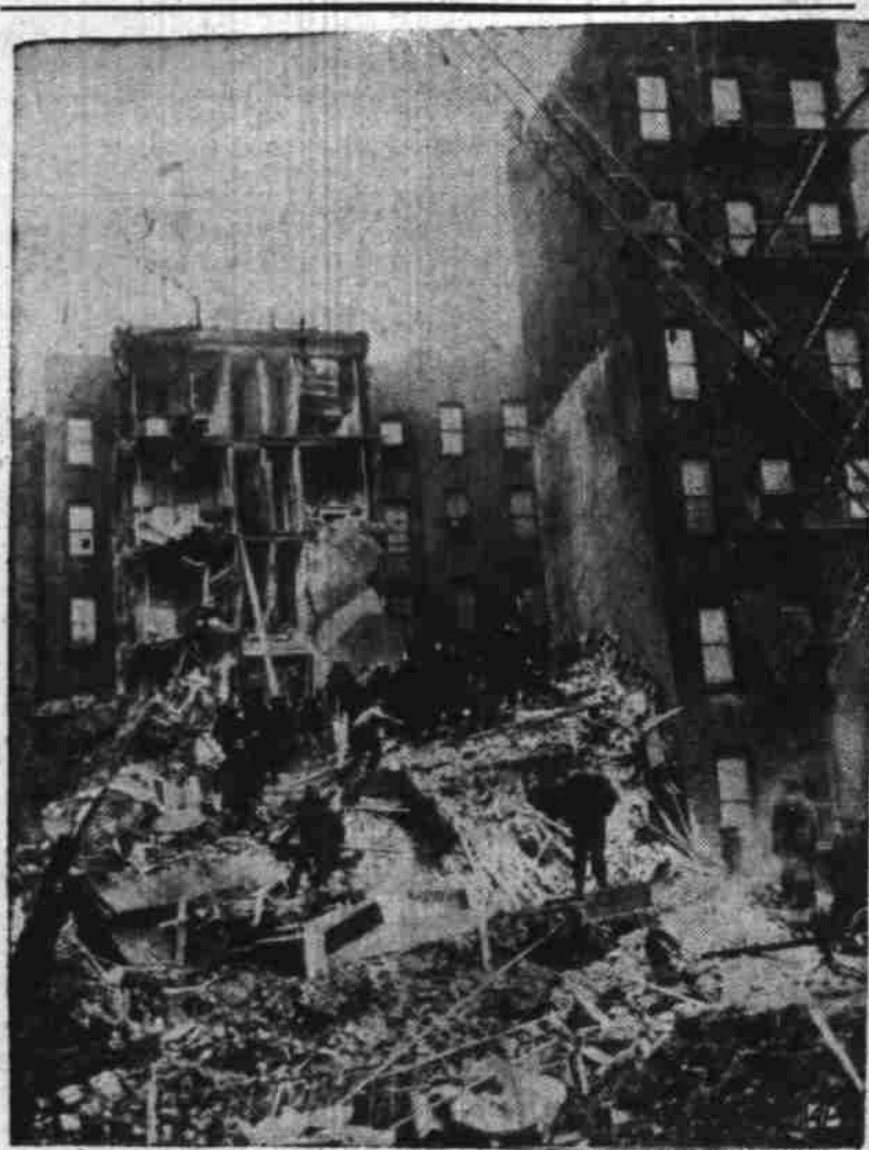
BLAST RUINS SEARCHED —Firemen aided by a big mobile crane (boom at right) dig through the ruins of a tenement which was wrecked by an explosion in an adjoining building, an ice house (debris in foreground), in New York. At least seven persons were killed in the explosion and subsequent collapse of the structures and about 40 others were believed missing. (AP Wirephoto).
