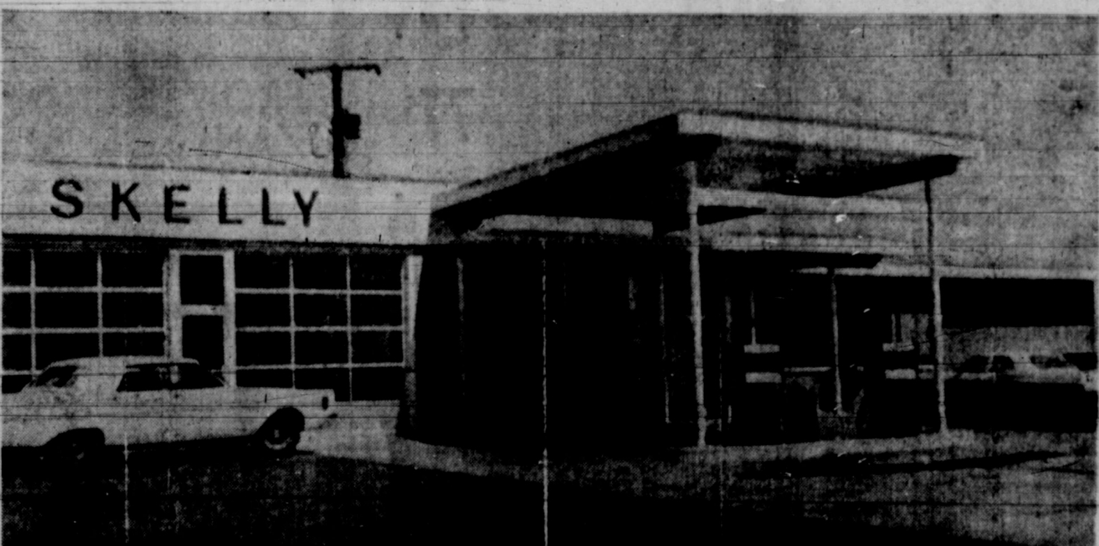
New Station And Cafe On Freeway
