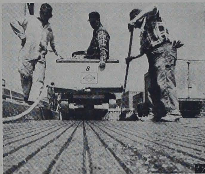
Machine equipped with a diamond cutting bar slices narrow grooves in roads where cars tend to skid in wet weather.
