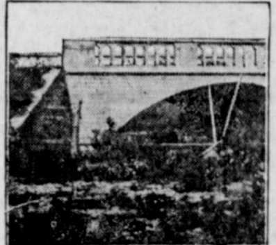
Skewed-Arch Bridge Used for Stream Crossing Road Diagonally—Note Position of Railing on Opposite Sides of Road.
