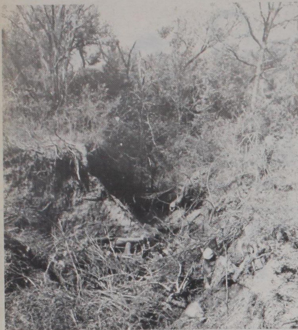
ABOVE, a critical washed area pictured in April before shaping. At right, the restructured waterway to be planted in Bermuda grass later this year.
