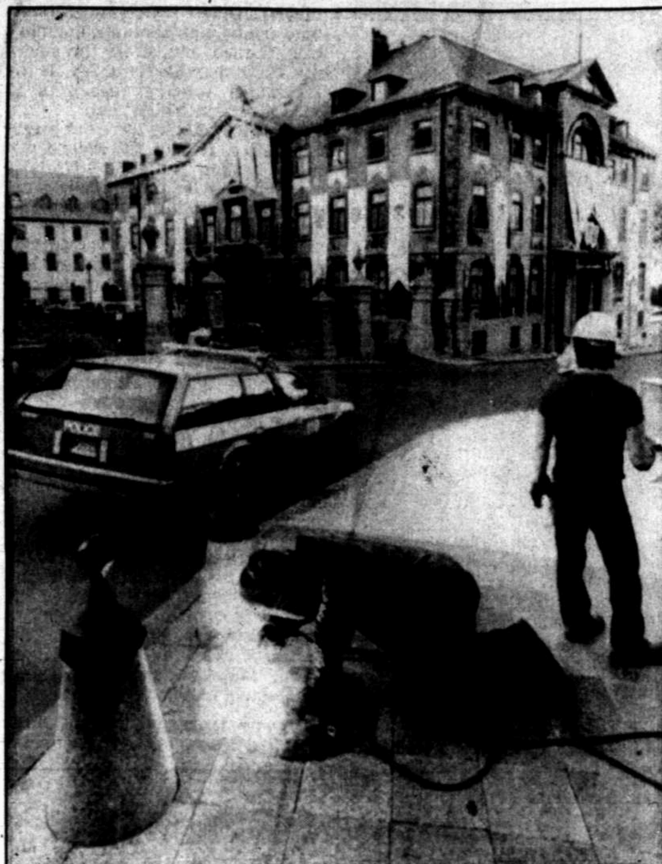
A Quebec city worker welds shut a manhole cover, a security measure in preparation for a papal visit.
