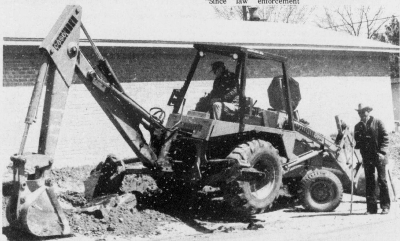
THE GROUND is being prepared for curbs and retaining walls around
