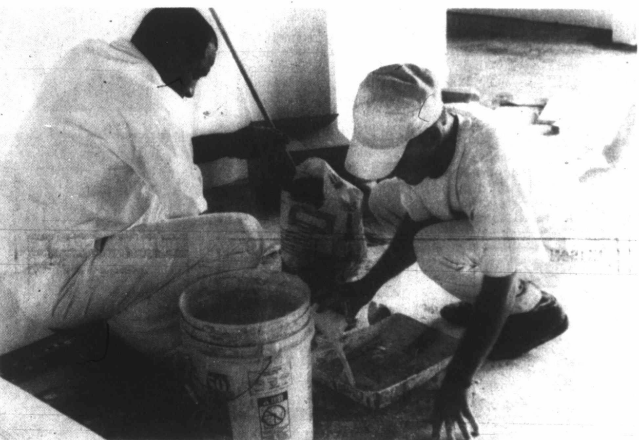
WALLACE UNIT inmates renovate the old Ed Lee Building on South Hwy. 208 for the opening of the new Boll Weevil Eradication district office. The business is expected to employ 35 people in the local office.
