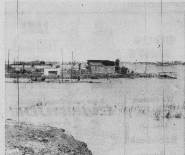
CABINS in groups and in isolated spots dot the entire shore line of Lake Thomas. Many of the cabins are modern permanent structures while others are move-in houses.
