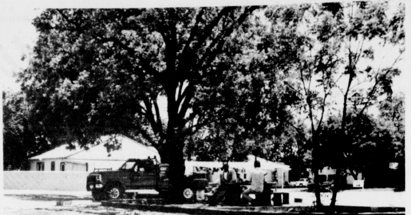
RENOVATION UNDERWAY —Workers take a break during work being done on the lot across from Winters Funeral Home. Purchased by the Winters Funeral Home Corporation (Ellen, Tim and Mike Meyer; Theresa Patterson; Linda Dry; Ray Alderman and Hattie Belle Bishop), the lot is being renovated for use as additional Funeral Home parking space. There will also be an area, equipped with picnic table, with a park-like atmosphere where families can relax. Levelling and landscaping has been done to enhance the trees and picnic table, which were acquired with the lot. A house which was on the lot was torn down approximately one year ago.
